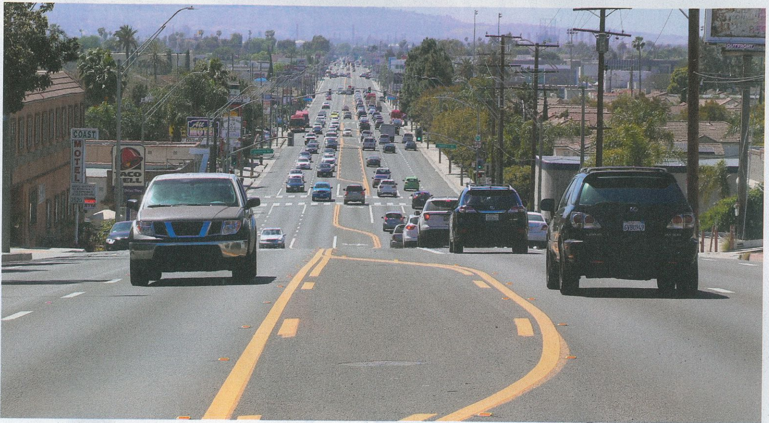
The 22-mile stretch of the Pacific Coast Highway serves as a vital arterial roadway for Los Angeles County, carrying more than 70,000 vehicles per day, spanning to a width of 7-8 lanes and consisting of more than 130 lane-miles of pavement surface. It services a diverse group of users and has tens of thousands of businesses within immediate proximity of its travel lanes.
