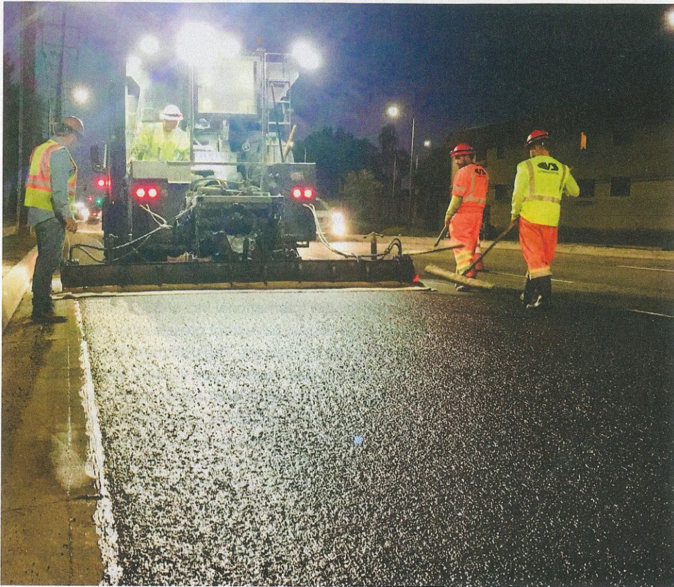
The treatment chosen for this section of Highway 1 was a Type III slurry seal application, which due to its being coarser allows for a heavier application rate that will help address and correct more severe surface defects and improve skid resistance under very heavy traffic loads.
