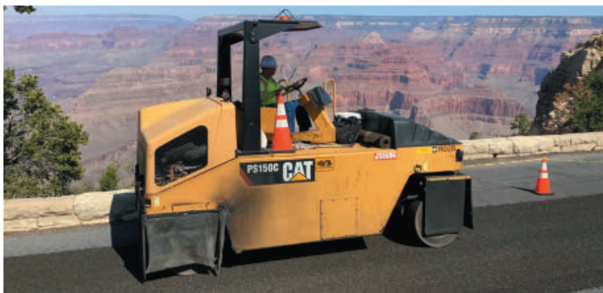
Pneumatic roller seats aggregate in chip seal above Grand Canyon
