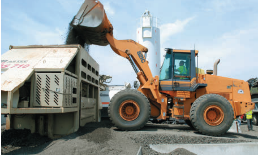
Millings from Virginia I-81 are placed in hopper feeding KMA 220i plant in CCPR operation
