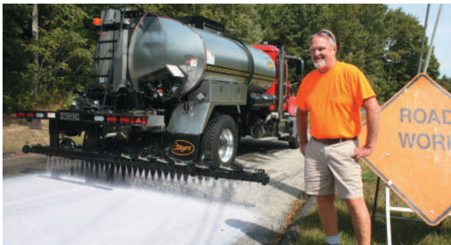
John Navarro, public works director of Town of Woodstock, Ct., oversees application of Delta Mist rejuvenating fog seal by Etnyre distributor operated by Riverside Asphalt Services
