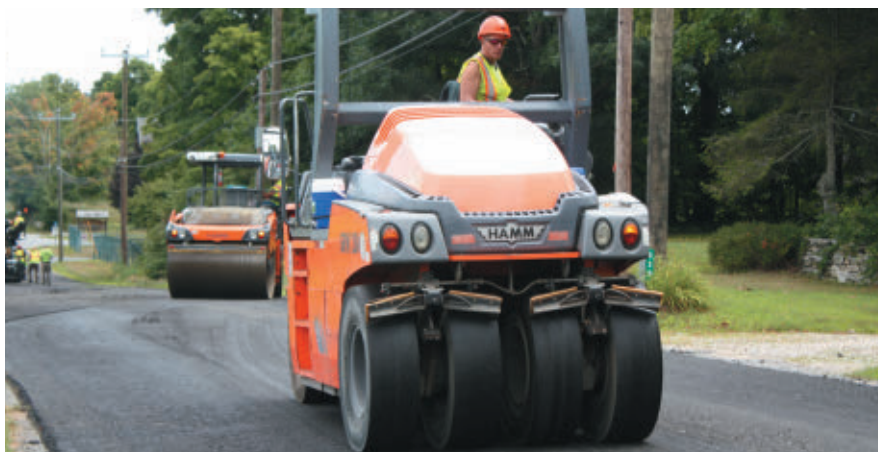
In Town of Woodstock, Ct., cold in-place recycled (CIR) lift is compacted with Hamm GRW 280 rubber-tire roller (right) and Hamm HD 120i steel-drum vibratory roller (rear)
