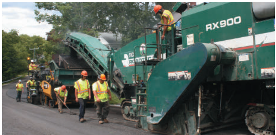
In CIR operation, Roadtec RX900 recycler/cold milling machine supplies a Caterpillar AP1055F paver with cold recycled mix that has been replenished with emulsion and will serve as stabilized base for double chip seal
