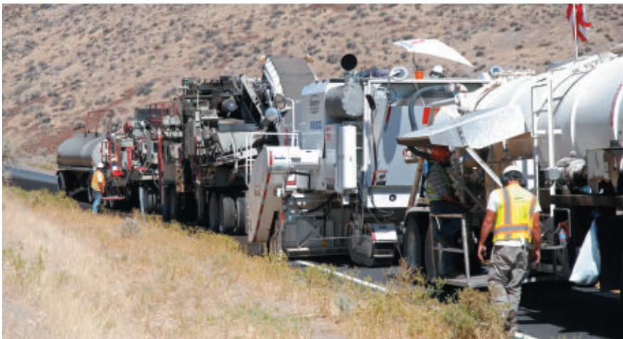
In Nevada, Washoe County road gets cold in-place recycled (CIR) via recycling train, eliminating long hauls of both recovered material and virgin hot mix asphalt
