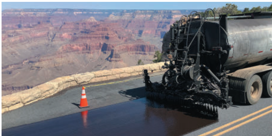
Emulsion placed in Grand Canyon chip seal
