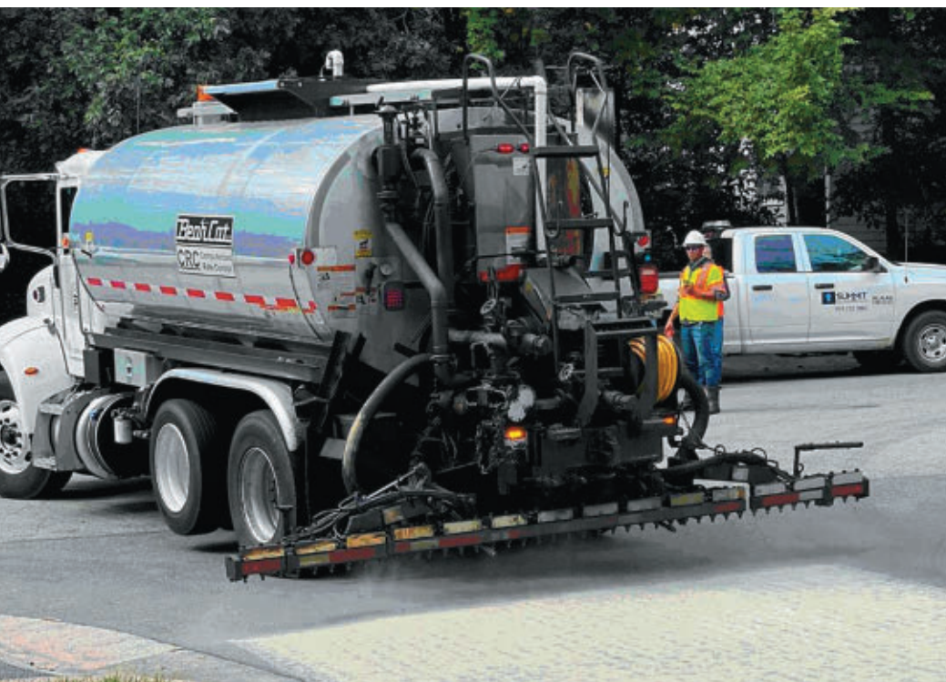
PTI's PlusTi™ asphalt rejuvenator/sealer application, Raleigh, N.C., 2020
