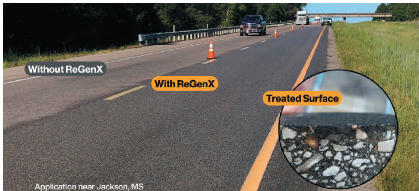
Near Jackson, Miss., regenerator-treated lane is contrasted with untreated lane
