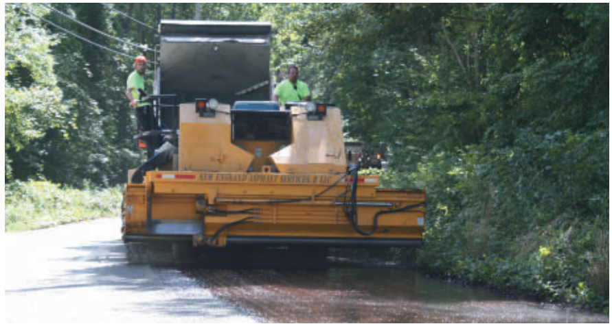
New England Asphalt Services' Etnyre chip spreader drops chip seal aggregate as part of town's autumn asphalt pavement preservation program
