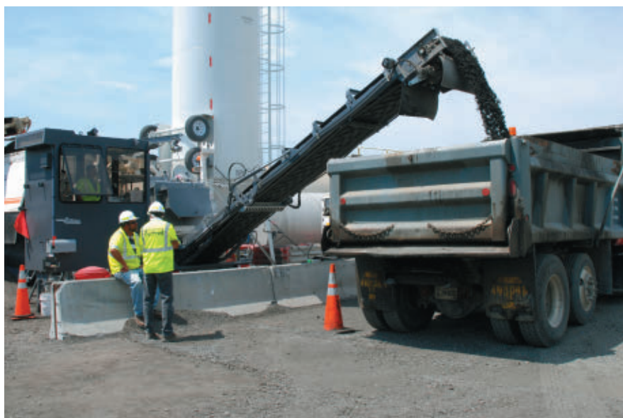
In Virginia, at nearby interchange, millings from pavement of I-81 are foam-recycled in portable Wirtgen KMA 220i cold central plant mixer and are trucked back to project for placement as base
