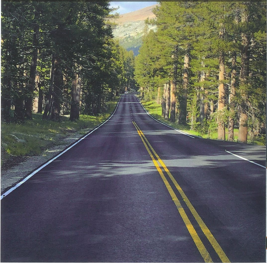
Below: Type III microsurfacing on Tioga Road Near East Gate - elevation 9,632 feet.
