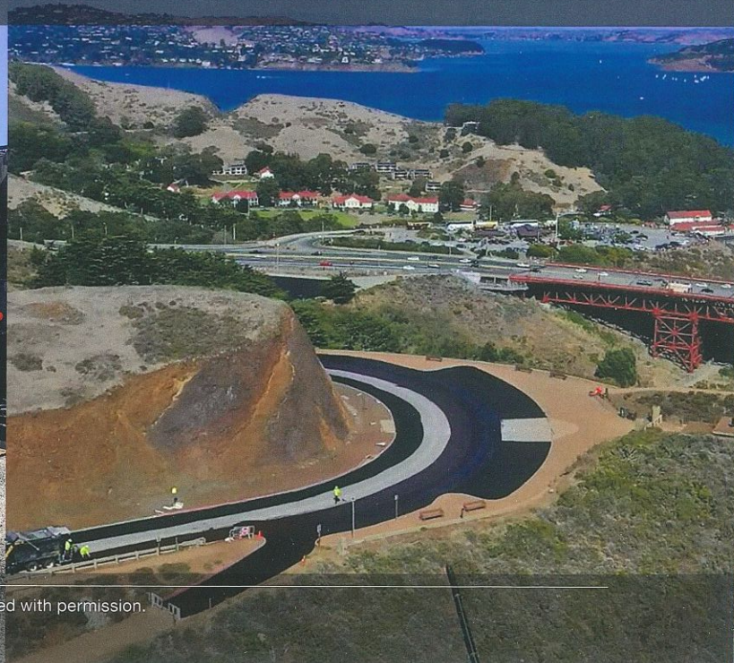
Below Left & Right: Type II microsurfacing being applied at the East Conzelman Road mainline and all parking areas.
