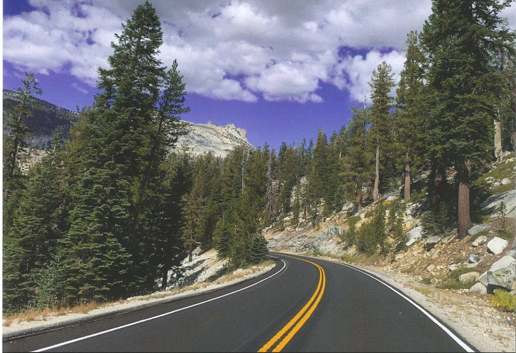
Above: Type III microsurfacing finished product on Tioga Road - elevation 8,530 feet.
