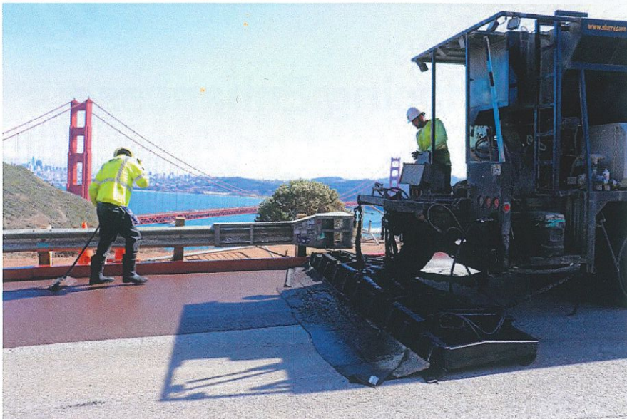
Hand work assures quality placement of micro surfacing
