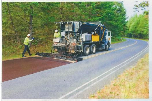
to be addressed prior to the preservation treatment as a slurry seal will not repair structural failures. Therefore, prior to any slurry seal being placed, areas of failure were removed and replaced with new hot mix asphalt.
