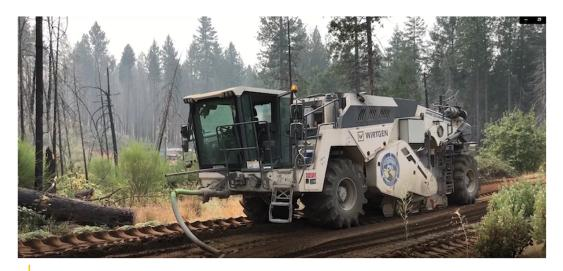
Pavement Recycling Systems pulverizing Jesus Maria road with a Wirtgen WR 250i cold recycler. The pulverization process includes the mixing of cement and water with existing asphalt and base to a depth of 9 in.
