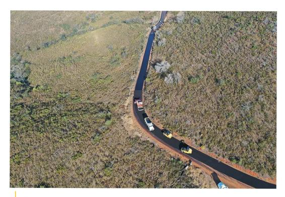
VSS International crews performing chip seal treatment to Jesus Maria Road. An oil spreader sprays polymer modified CRS emulsion to the roadway followed by an application of 3/8-in. chips with pneumatic tire rollers behind the chip box to lock in the chip seal treatment.
